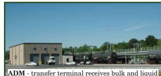
ADM - transfer terminal receives bulk and liquid processed agricultural commodities in hoppers and tank cars. These are transferred to trucks for delivery to the end user in the local area.
